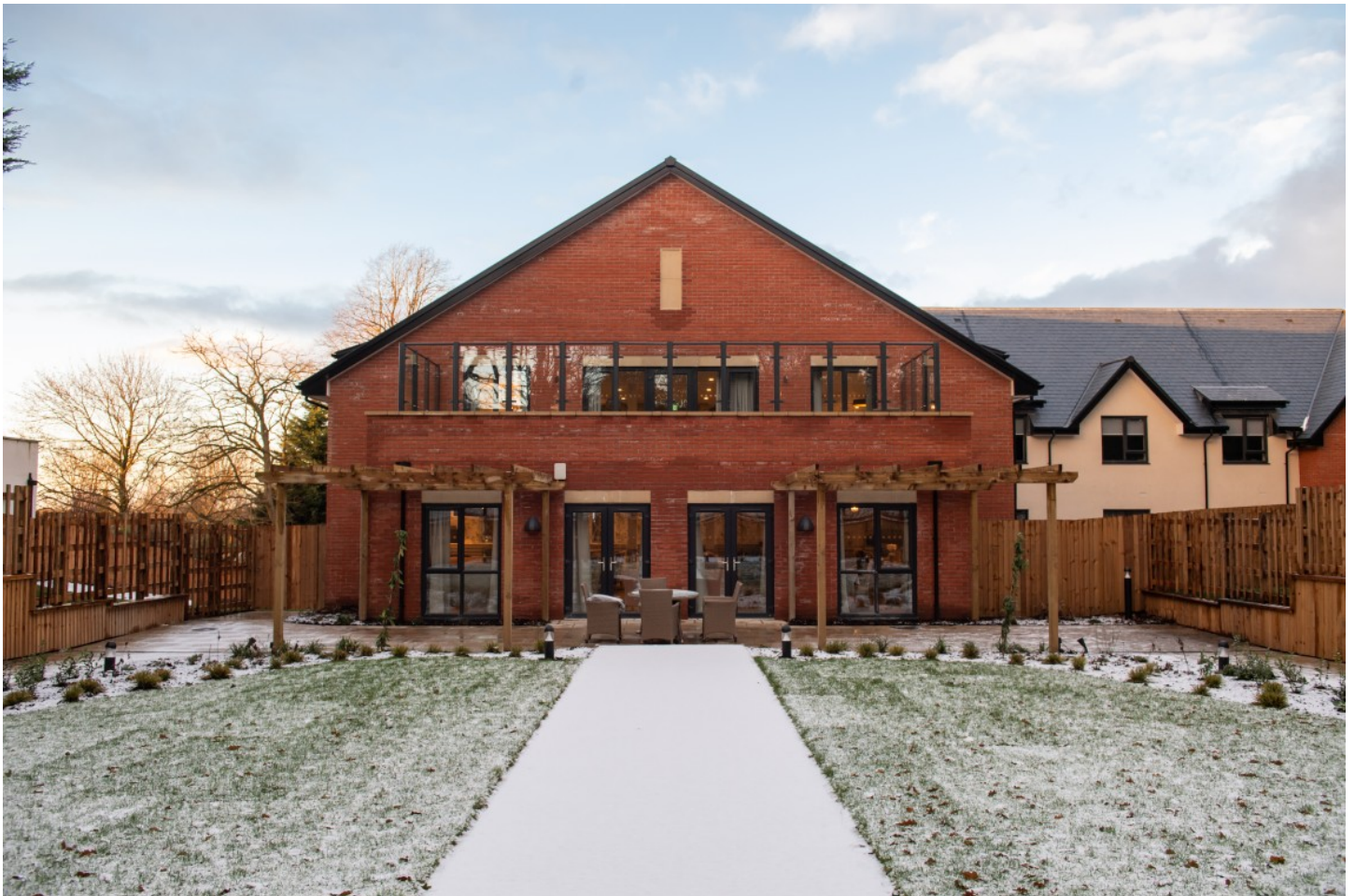
Intergenerationele community Lymm. Foto ©McGoff Group
